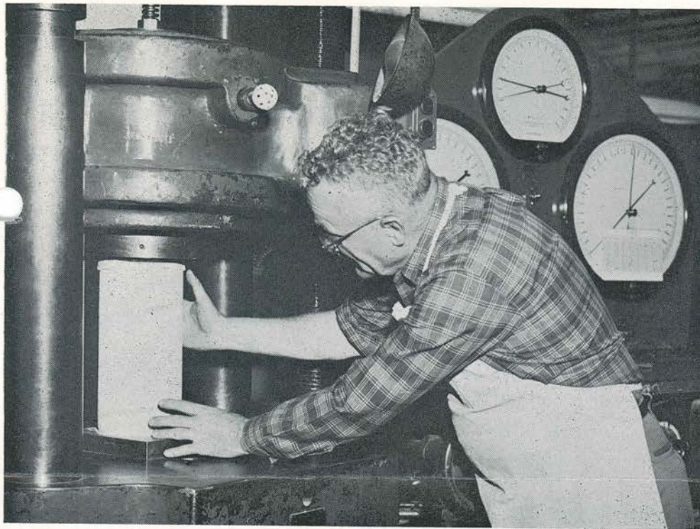
SCOTT H. HUNTER retired on February 28 as a road materials inspector for the department of applied mechanics after 45 years of service. Hunter inspected this concrete sample for a Kansas contractor on his last day of work. This materials testing machine is being replaced by a new $42,000 MTS shown elsewhere in this issue of IMPACT.
