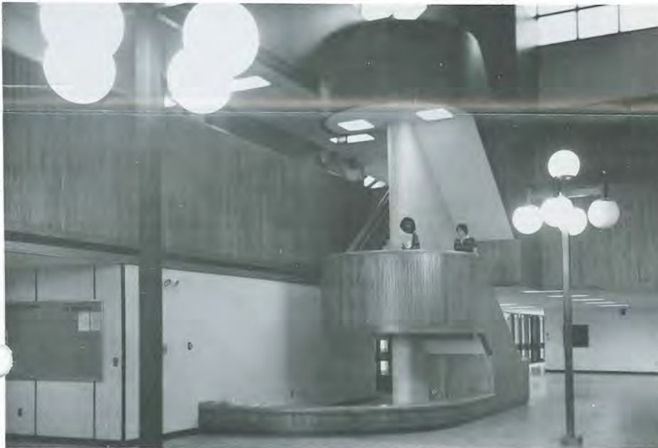
Plants, artwork and even a pendulum soon will grace the vaulted, three-story atrium of Durland, Phase II. The pendulum base is being constructed by Kansas State University artisans, with the pendulum design by engineering faculty. It is expected to be in place for dedication ceremonies.
