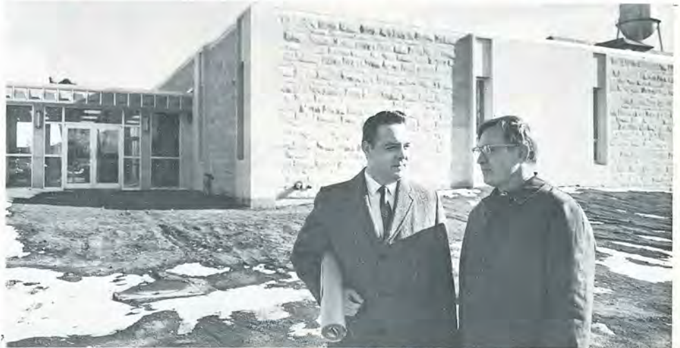
WEST SIDE VIEW of the new $900,000 addition to Ward Hall housing the department of nuclear engineering. Faculty and staff will move into the new facility in two or three months, says Dr. Richard E. Faw (l.), professor. Faw is shown with Ray Lippenberger, a K-State architect. Ward Hall houses the KSU Triga Mark IV teaching-research reactor.
